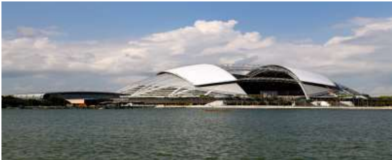
Singapore national stadium's moving roof.
